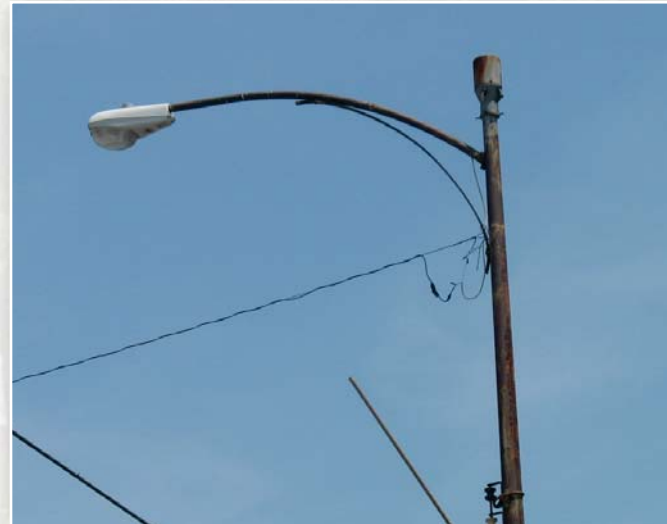
Here is an example of the current lighting fixtures found throughout Boonville.
