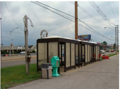
raised platform to distinguish the boarding area. The plastic panels on the shelters are almost opaque and need to be replaced with tempered glass; at one time it appears that the shelters were illuminated with advertising since there is an old electric service panel nearby. Due to the number of passengers boarding at certain times, three passenger shelters are most likely required.
